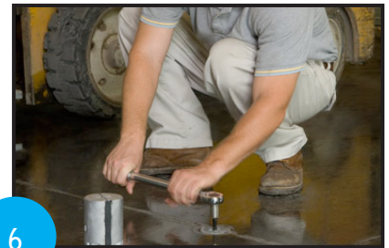
SD Joint Stabilizers are expanded by torquing to 85 ft. lbs.
