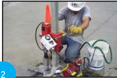
Certified installers use specialized equipment to drill core holes.
