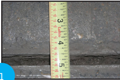
Survey slab, measure and record deflection (optional), determine location for installation and repairs.
