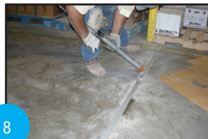
Additional grinding, filling and finishing may be necessary to complete the repair.
